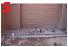
Install pavers or finish pavement surround to required level, should be 1/8" above grate.
