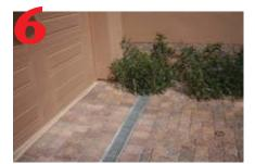
Clean away debris, remove protective plastic if necessary. Seal joints if required.
