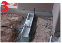
Lay channels starting at outlet. Set a string line at required height to ensure level.
