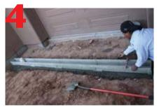
Continue to lay channels to required run length; continuously check alignment and level.
